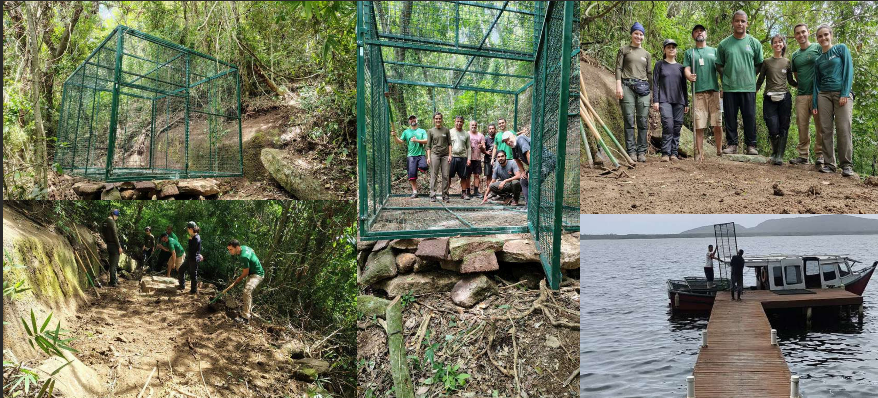
Instituto Fauna Brasil - Enclosure transport, site preparation, and installation. (Preparatory work for the 2027 wildlife rehabilitation program)
